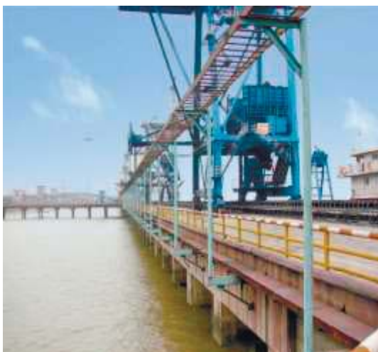
Fig. 2. Belt conveyors in Jiangsu Shagang Group
