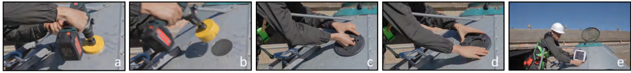
Figure 3: Three steps of the sensor installation procedure with (a,b) drilling, (c,d) adapter ring placement, and (e) sensor fixation.
