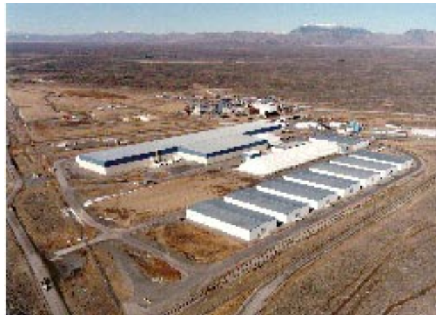
Figure 1: RCRA Compliant Storage Buildings
